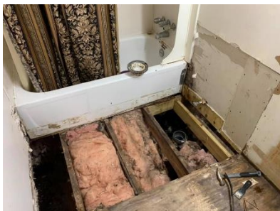
Pictured left: A rotten floor bathroom floor during mid-repair.
